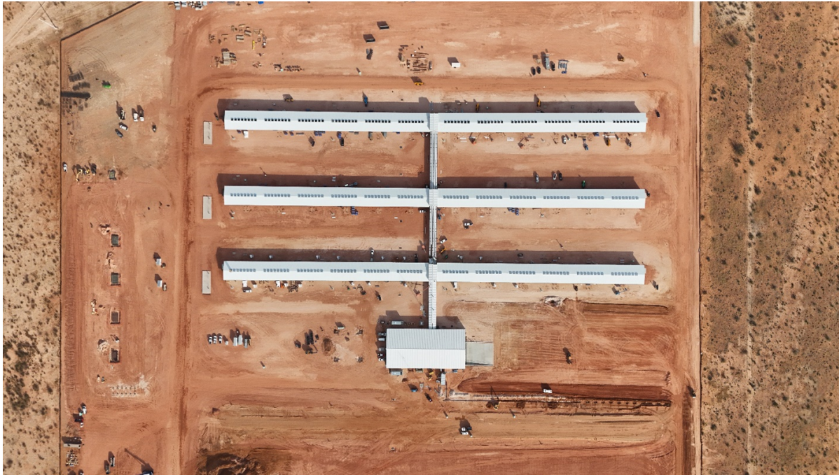
Construction at Black Pearl site
